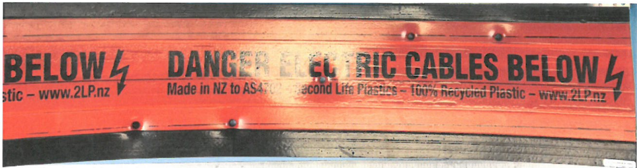
300mm cable cover after penetration test
